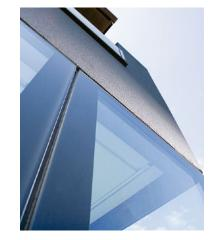
The special design: Structural Glazing The outside level provides a unified glass envelope. The glass joints are without profile at the outside and project clean modern lines.
